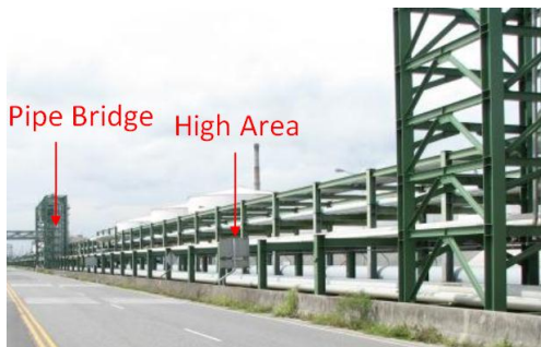
Figure1. The group of inspected pipeline.
